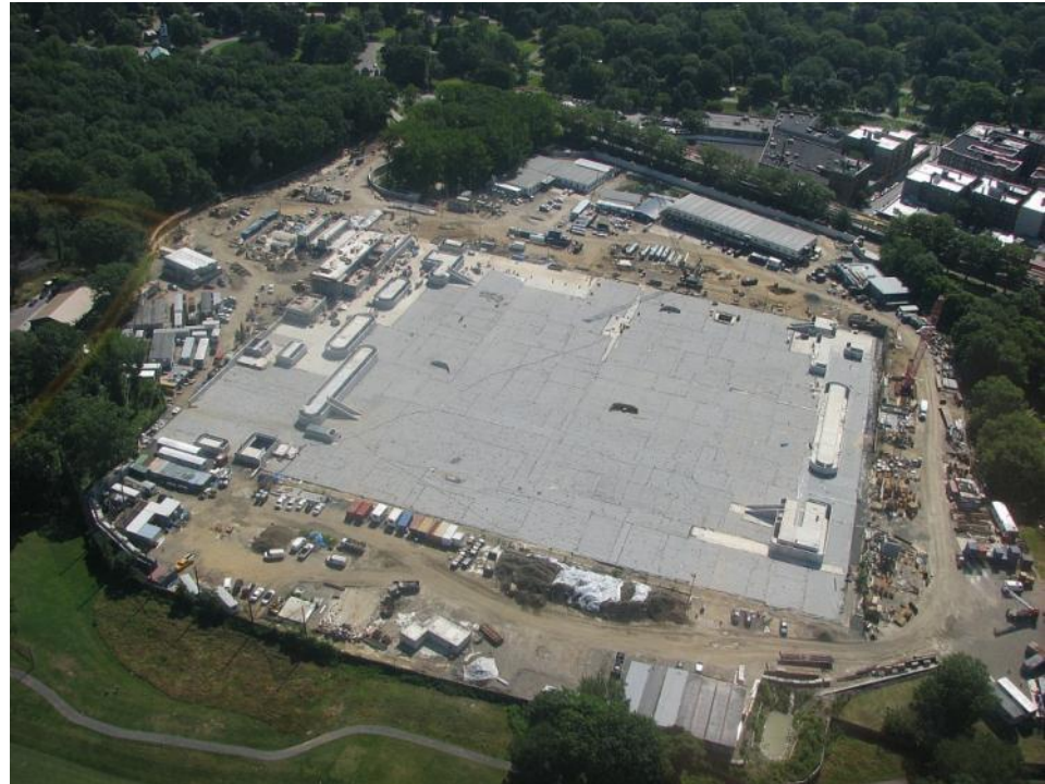
Croton Water Filtration Plant
