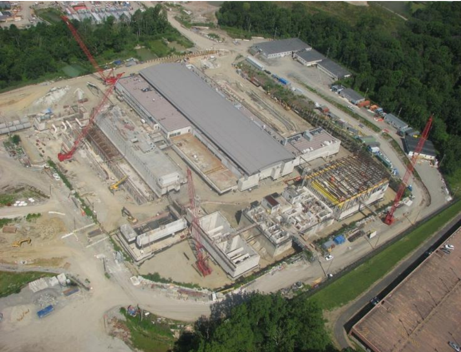
Catskill/Delaware Ultraviolet Disinfection Facility
